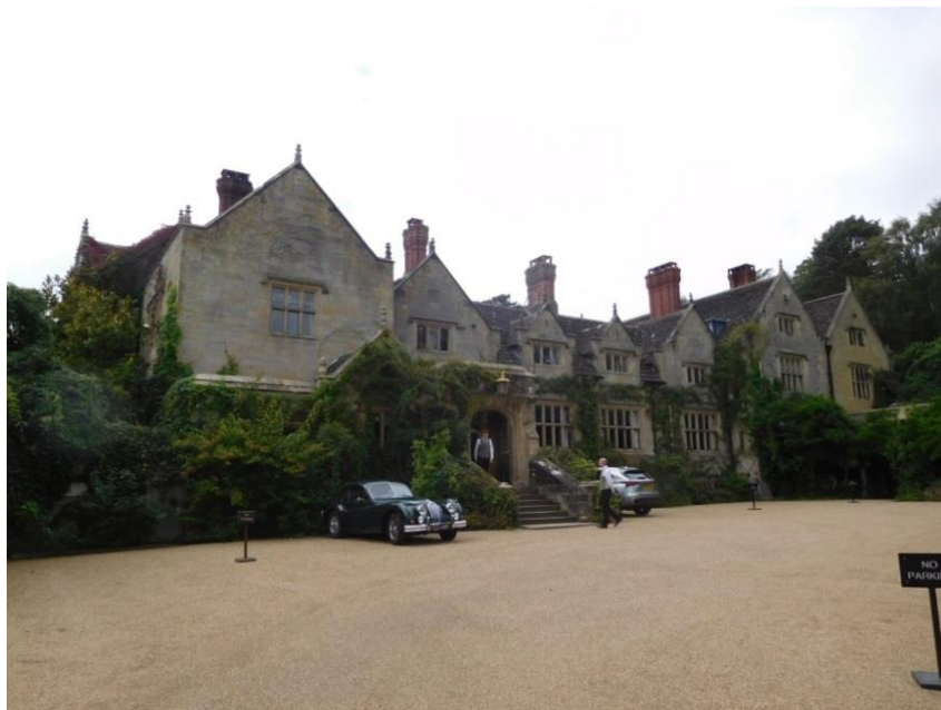
George & Peto wing with re-positioned front door. Two gables of 1992 extension on far right.
